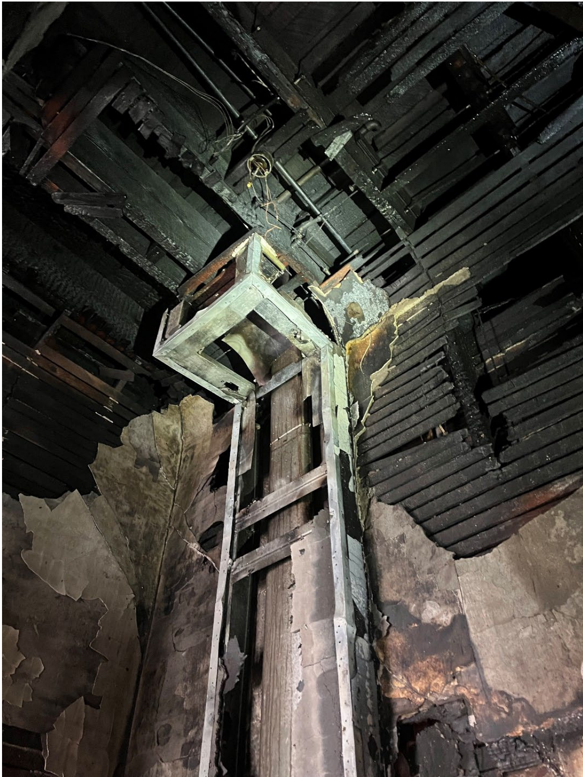
Old, inactive kitchen flue provides a space for fire to travel.
