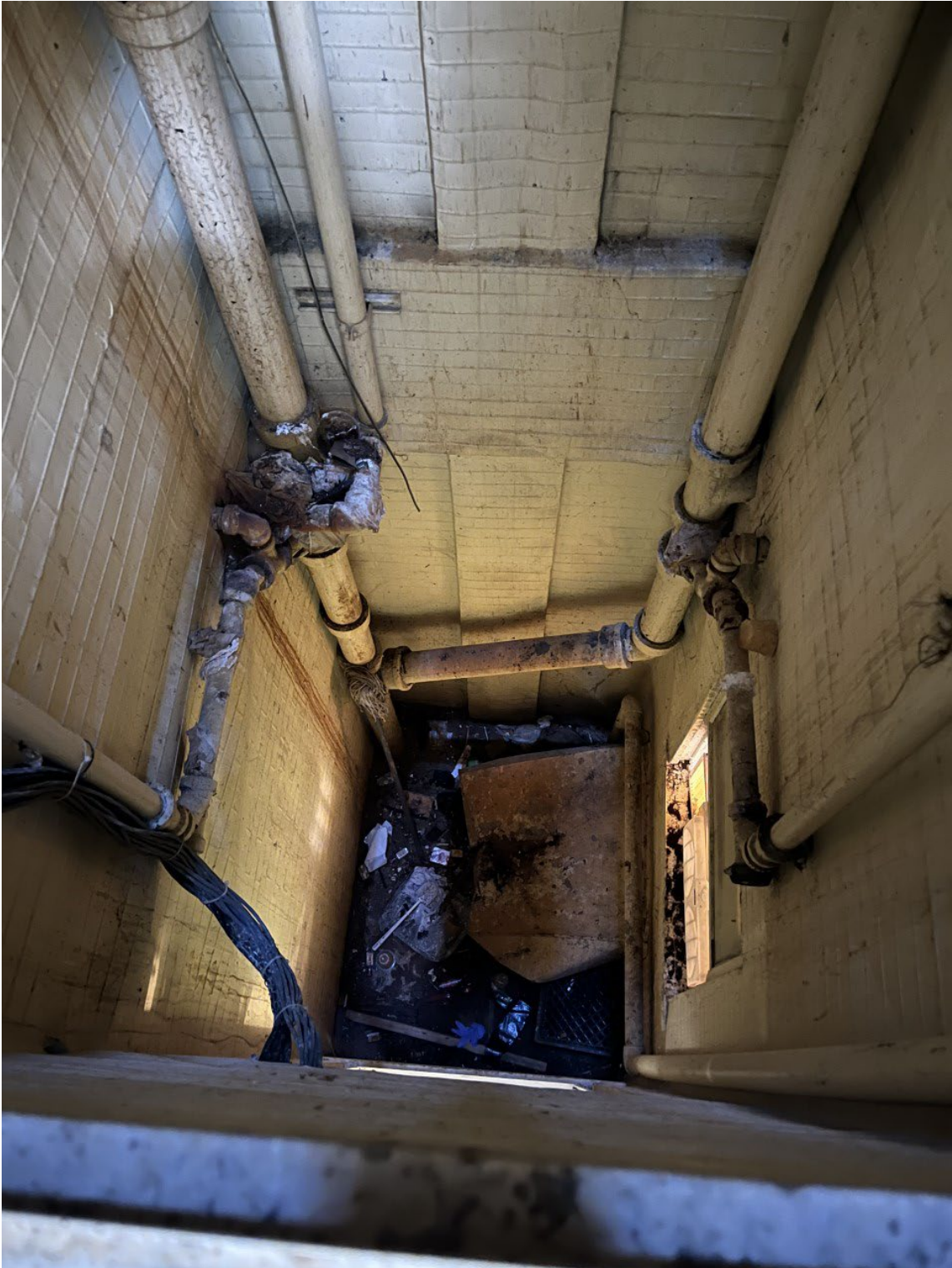
Discarded trash at the base and hung up on piping can be ignited by a discarded cigarette
