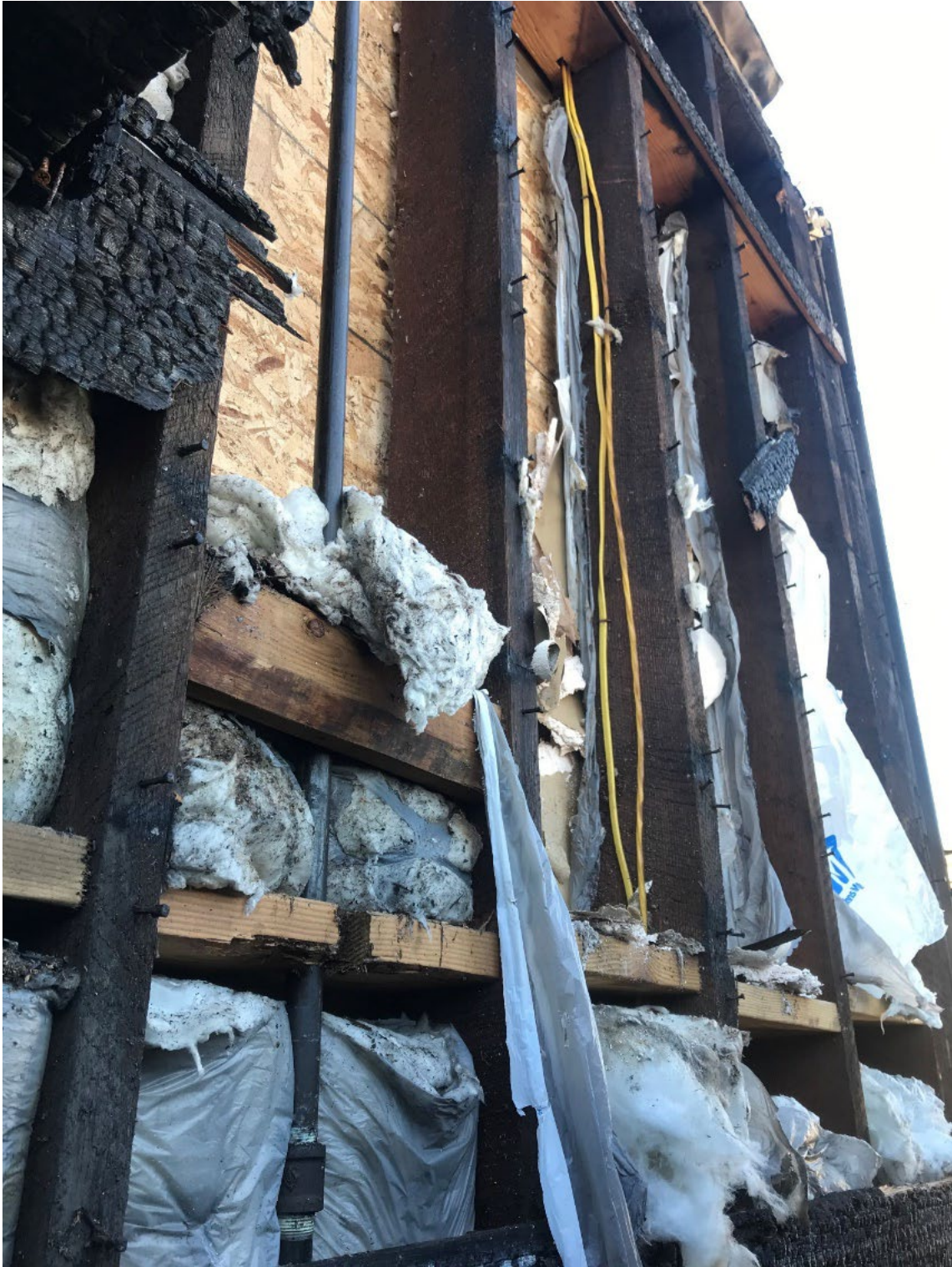
Exterior Walls opened due to presence of shear wall (1/2" plywood) on the interior. Notice Black pipe (gas) and Romex (electrical) as possible hazards.
