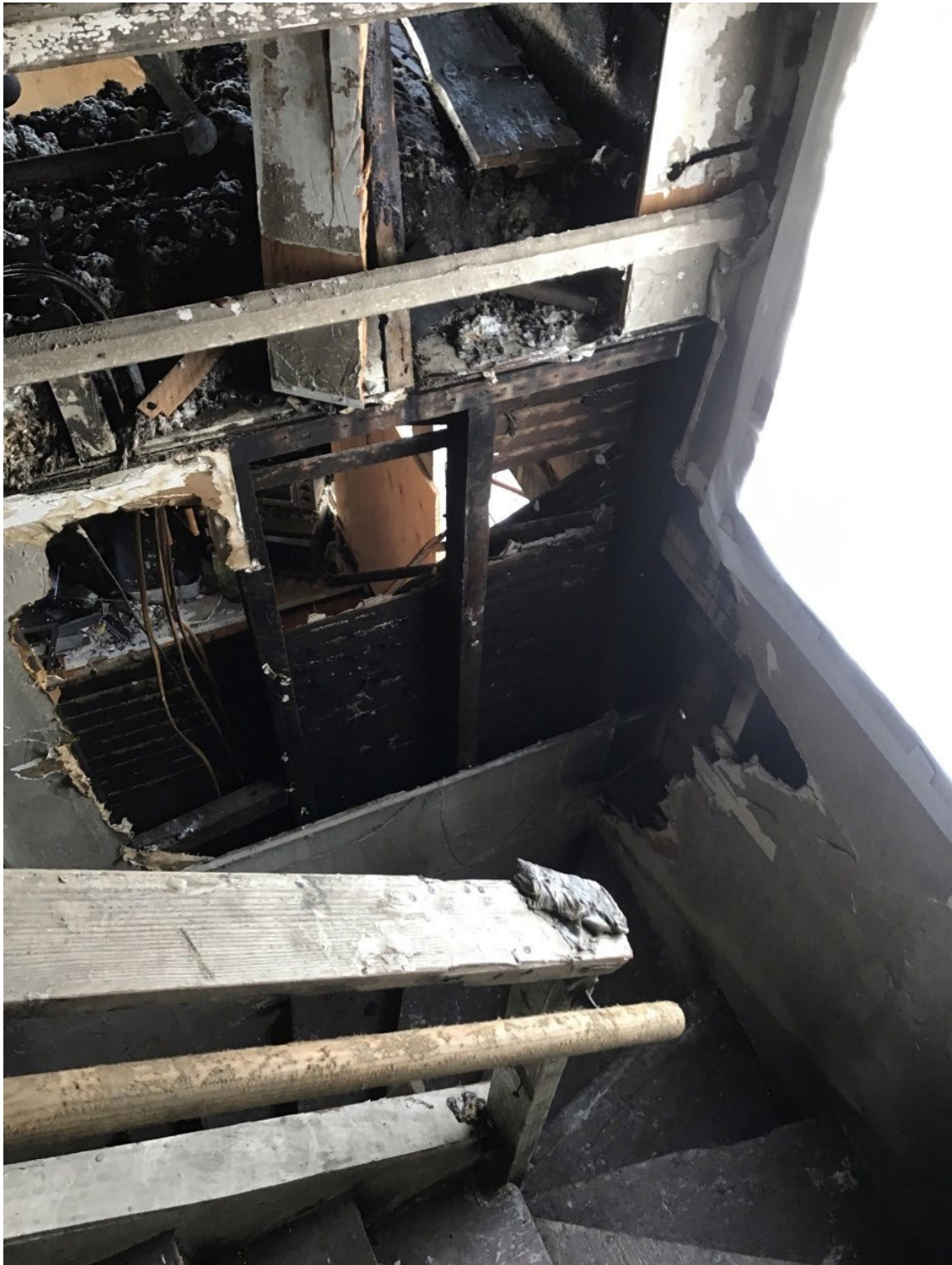
Accessing the attic from a stairwell: This tactic successfully employed to limit fire spread
