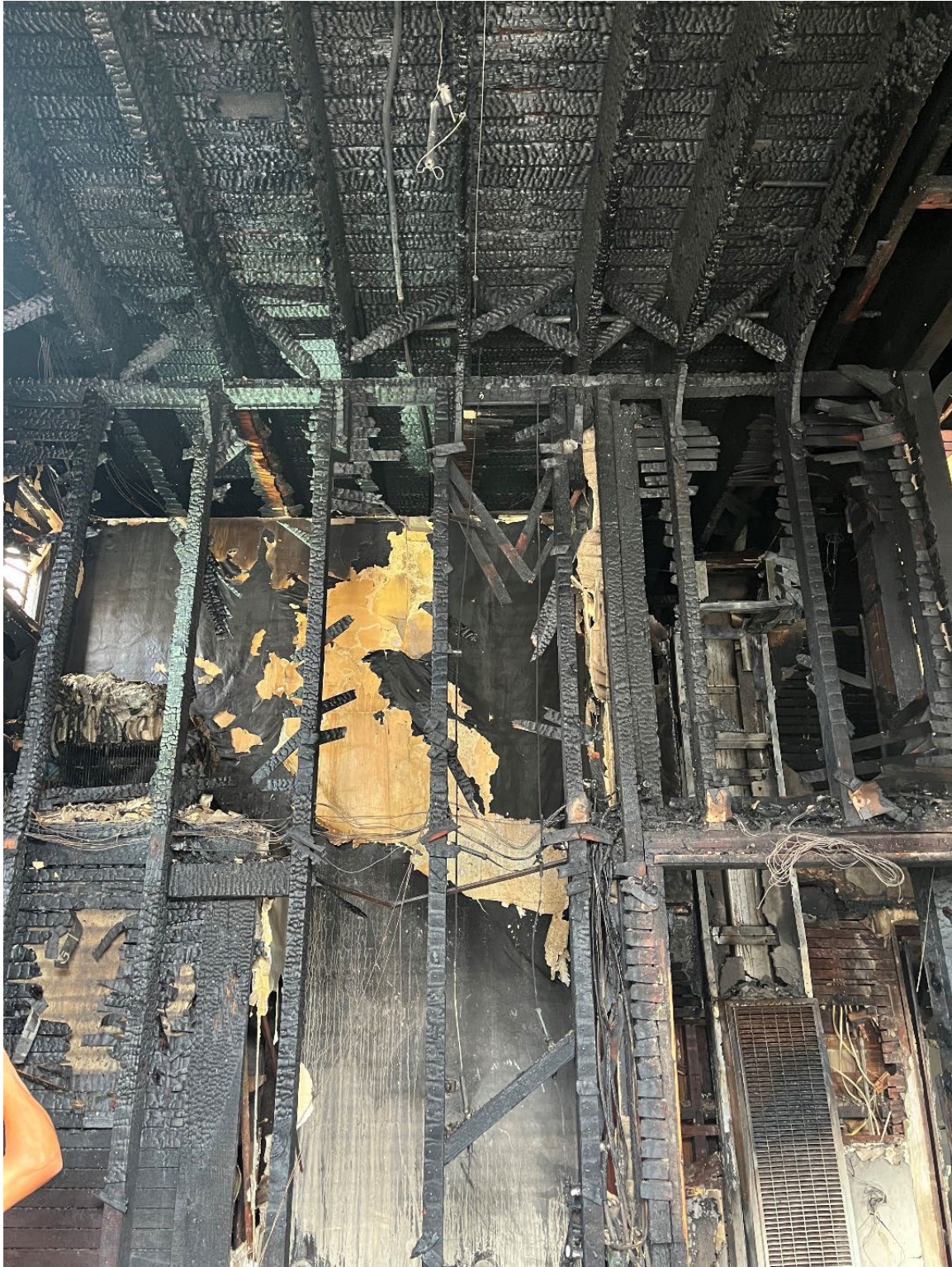
Notice bottom right wall furnace. The flue will run all the way through the attic and vent above the roof. This presents a path of travel for fire in the walls.
