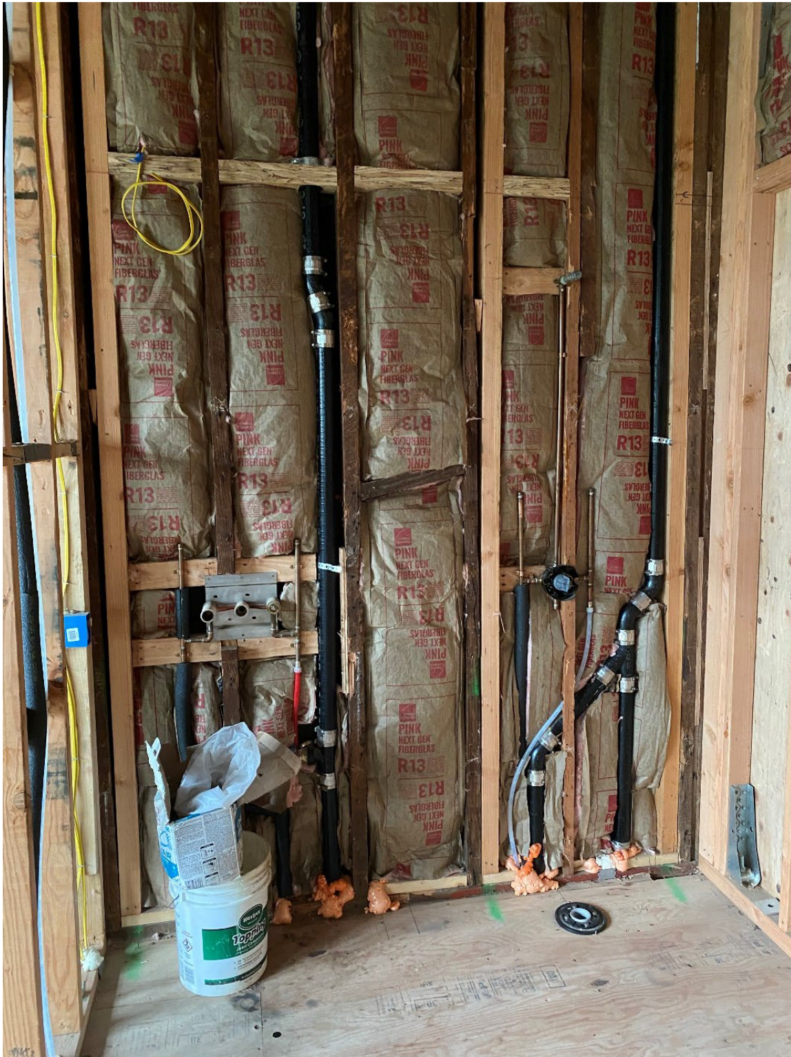
Common plumbing for bathroom shower and vanity. Notice the 2x4 blocks either penetrated through or removed (over the shower) for drain vents. This is where fire will travel.
