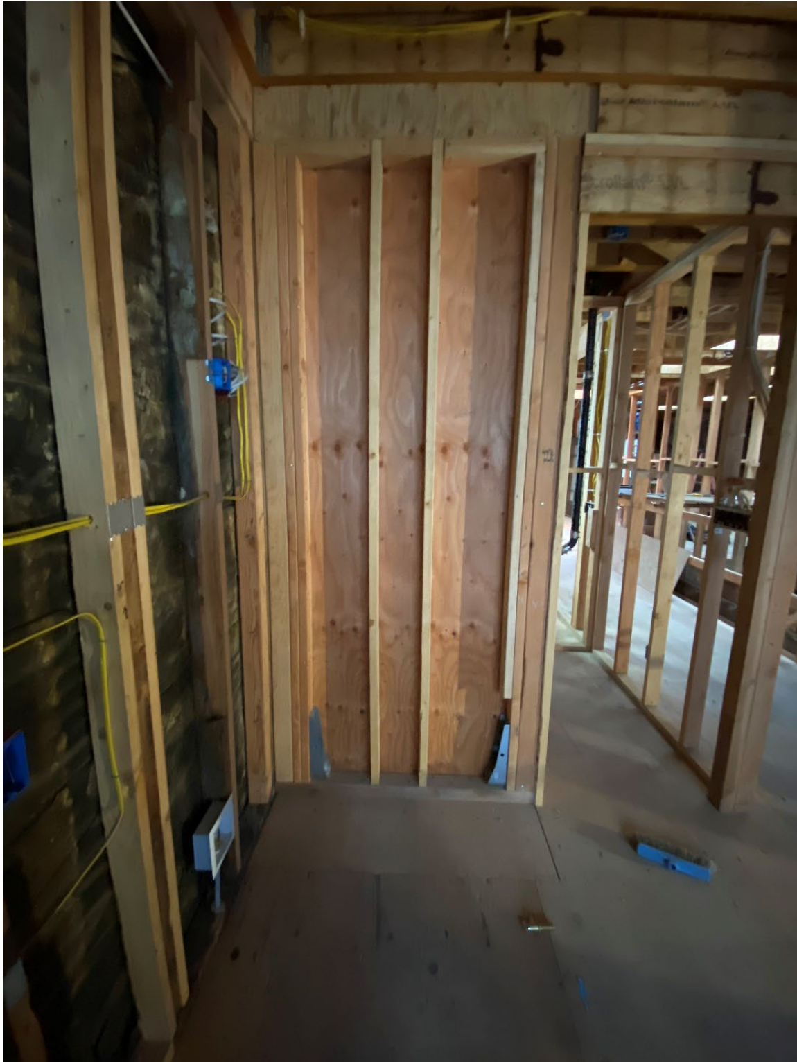
Interior Shear wall with Simpson hold downs. Identify the shear and do not cut near the hold downs. Also notice the nail plates to protect the Romex.
