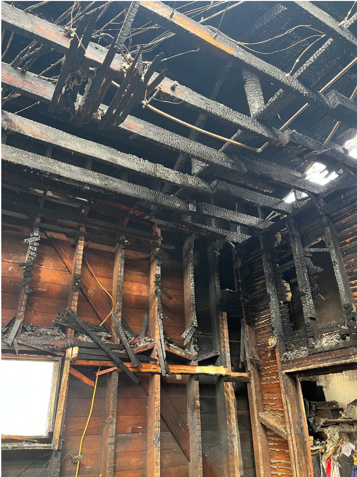
Note knob and tube wiring on the ceiling
