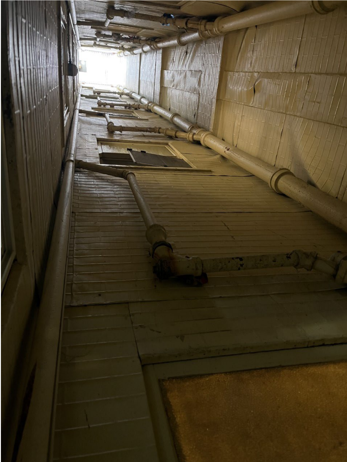
Notice the piping and sheet metal in this lightwell. Also notice the creases in the sheet metal where fire can enter the wall
